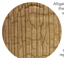
Alligatoring paint is paint that cracked in a pattern resembling alligator scales. This type of cracked paint makes a building look poorly maintained.
